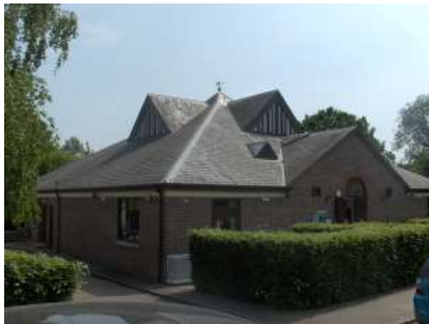
North Heath Hall, North Heath Lane.
