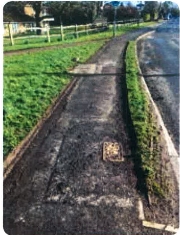
Case Study – Henfield Parish Council
