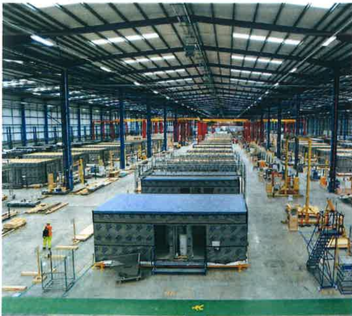
Factory Production CLT modules are produced in a safe factory environment
