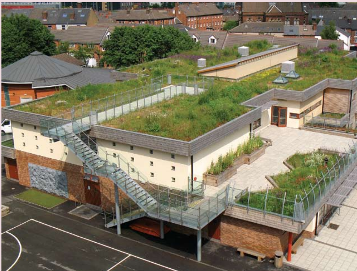
© Sheffield Green Roof Centre
